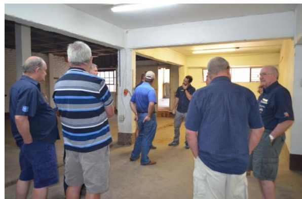
Inspection of Unit 55, Silverton Business Park.
